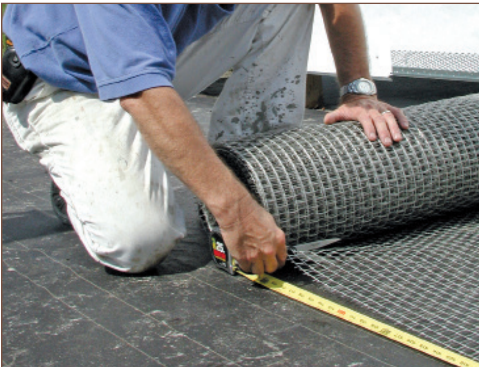
Figure 1 – Nonmetallic plaster bases cut easily.
